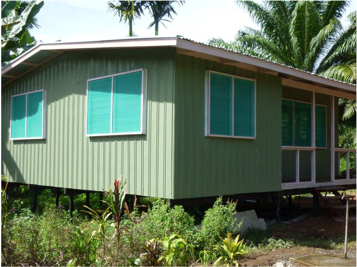
MBES Principal's House nearing completion yesterday 3-12-2014
